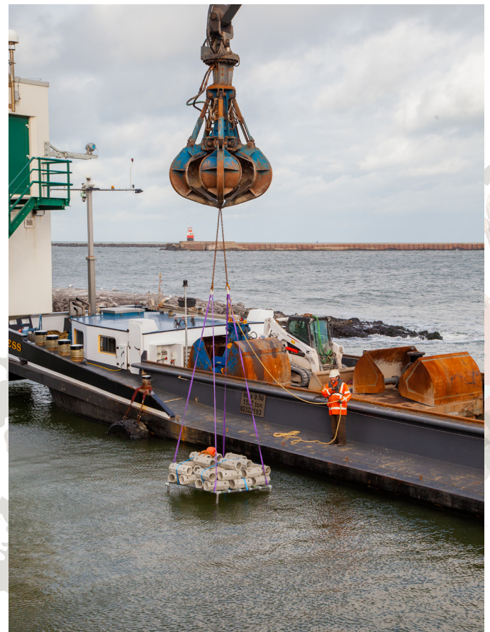
Reef installation in IJmuiden
